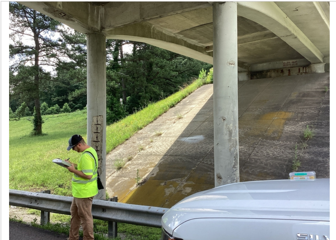
Bent #1 looking back
