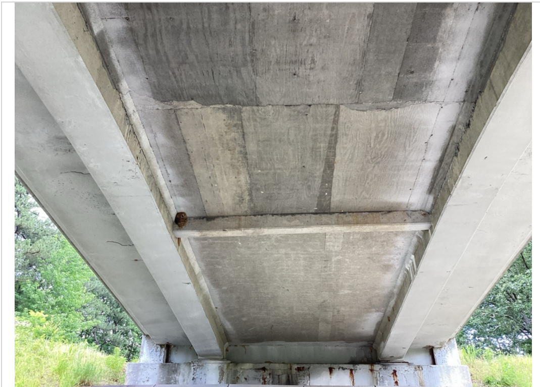
Bottom deck of span #3
