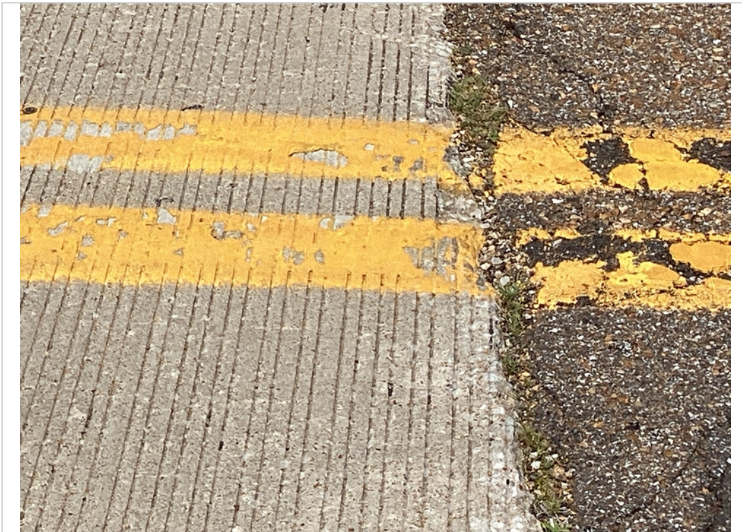
Span 3 spall
