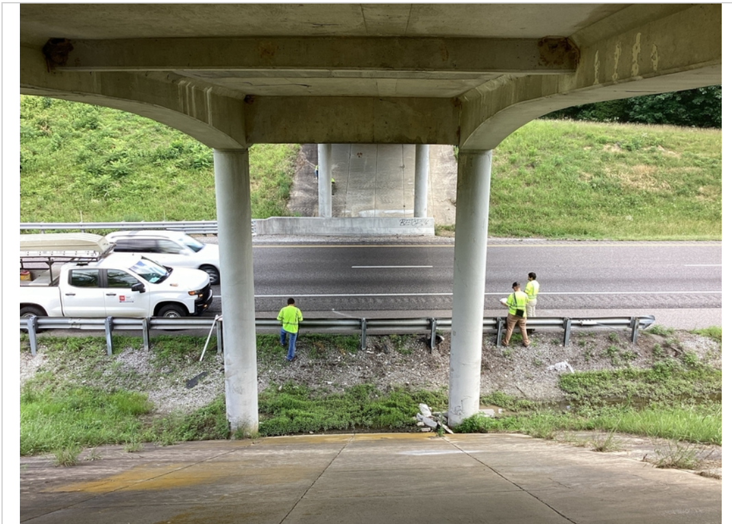
Bent #1 looking forward
